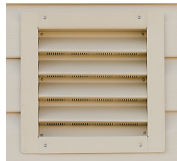
Gable Vent on Vinyl Shed
