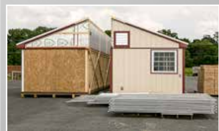
20x60 kennel comes pre fabricated in two 10' wide sections. Finished on site.
