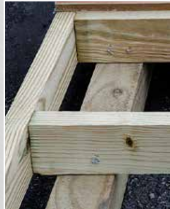
Pressure Treated 2x4 Floor Joists & 4x4 Runners
