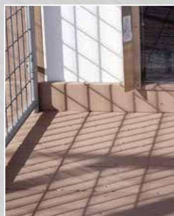
PVC Decking on Runs
